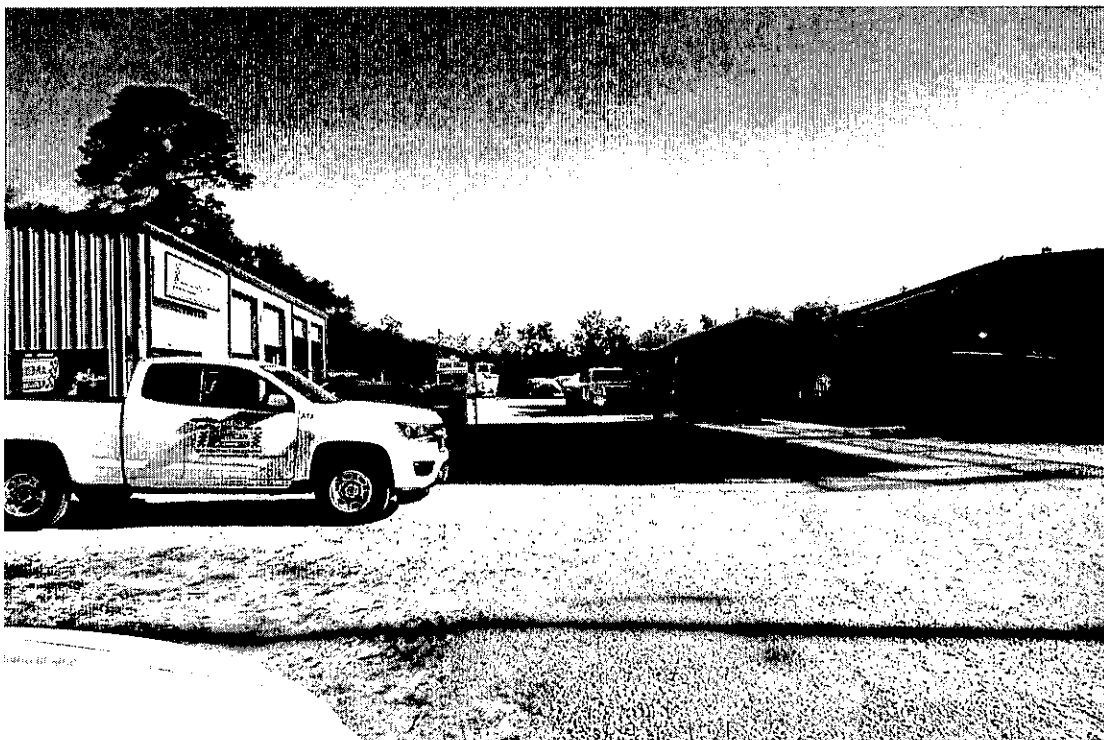
View toward service area.
